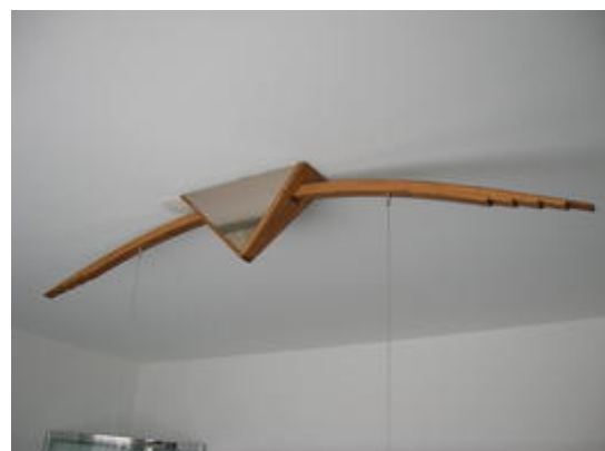
The transformer is hidden in here
