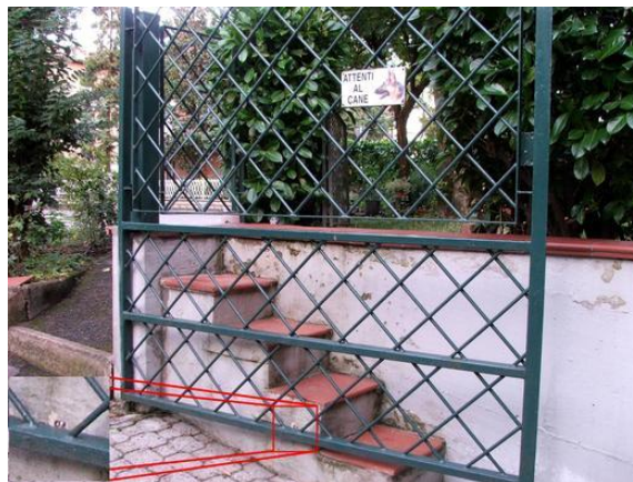
Opened gate with marked countersunk pot magnet
