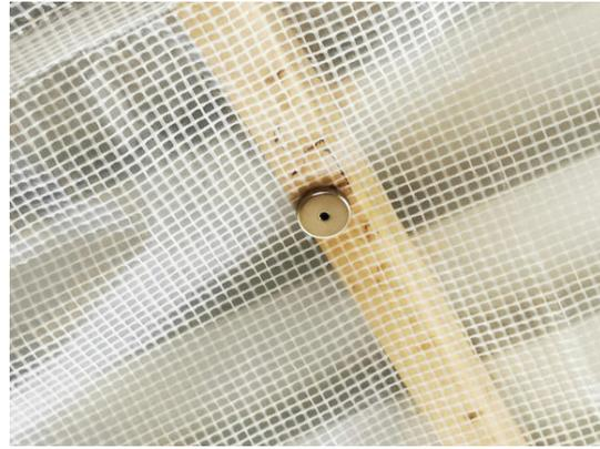
Sufficient for attaching the sheets to the ceiling surfaces: CSF-48 - ferrite pot magnets with counterbore ([www.supermagnete.de/eng/CSF-48](http://www.supermagnete.de/eng/CSF-48))
