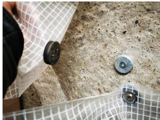
On the floor and in the entryway I used two galvanised 3 mm thick washers (hole: Ø 11,5 mm) each as counterpart for the magnet. Unfortunately, supermagnete.de does not yet carry these large stainless steel discs ;)
