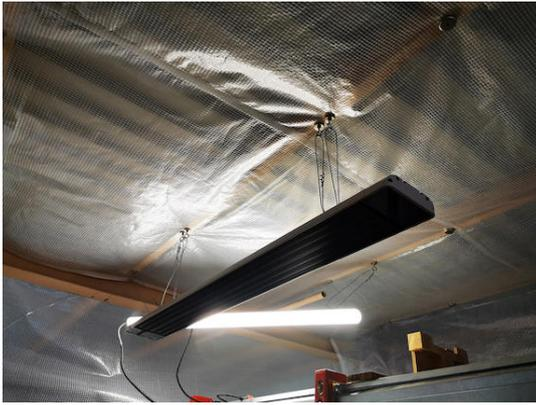
Ceiling fixture for the relatively heavy infrared heater: 4 of the OTN-40 - pot magnets with eyelet ([www.supermagnete.de/eng/OTN-40](http://www.supermagnete.de/eng/OTN-40))
